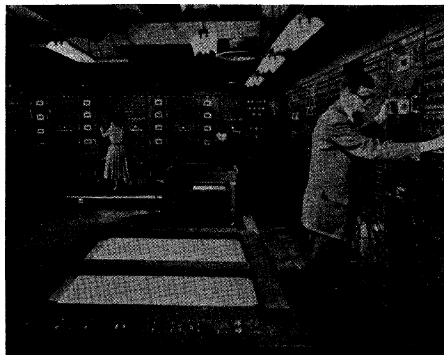
Figure 8—Reeves computer installation, courtesy Reeves Instrument Company
